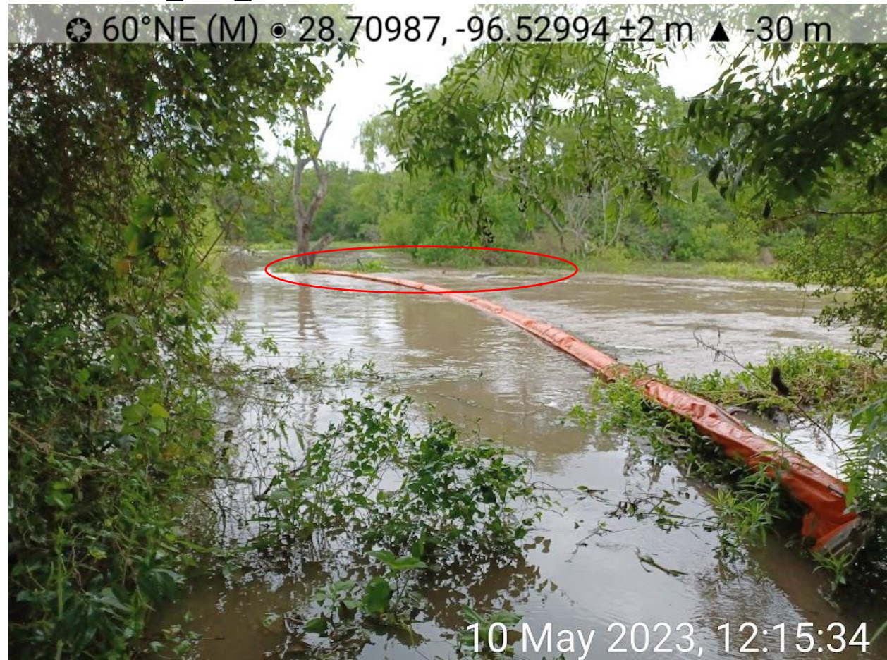
Boom that stretches across creek north of Outfall 014 had water flowing over top of it on the far side, in area highlighted by red oval.
